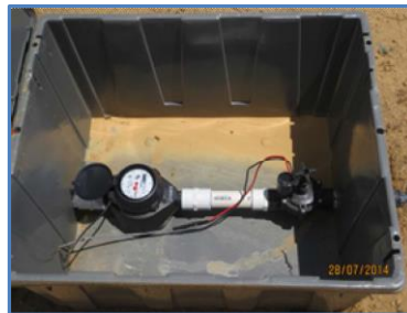
Fig 40b. Box with flow meter and solenoid at head of sensor-scheduled row.
