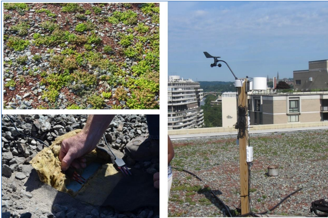
Fig 47. Green roof sensor network installed at Potomac Plaza, Washington, DC.
